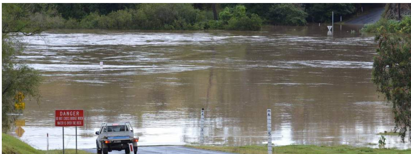
Photo: Toorooka Bridge
