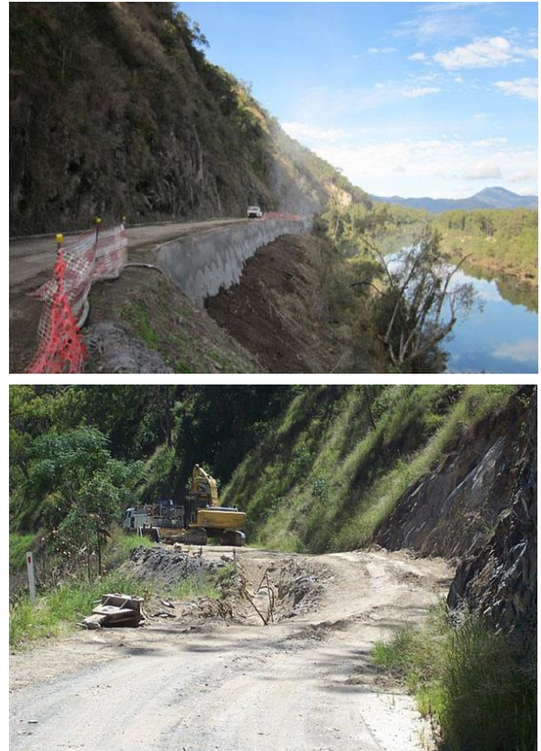
Figure 15. The Kempsey to Armidale Road
