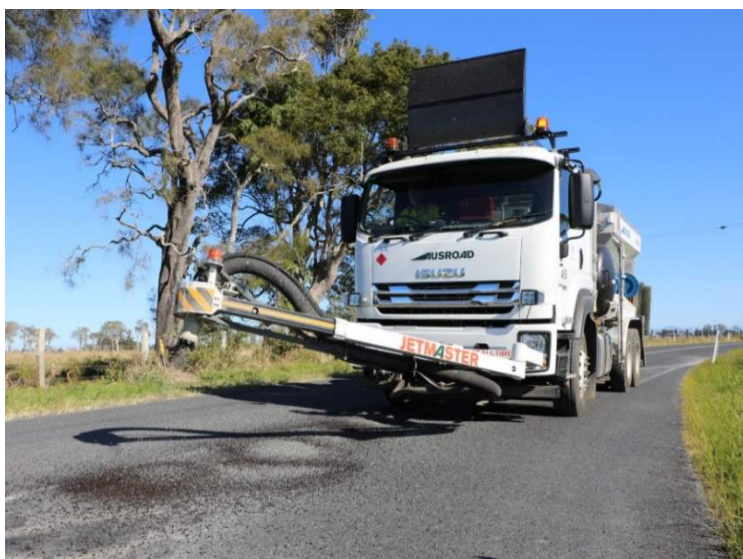
Photo: Council jet patcher
