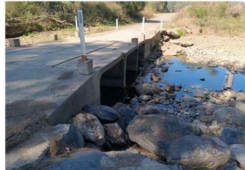
Photo 4: D/S Dungay Bridge
