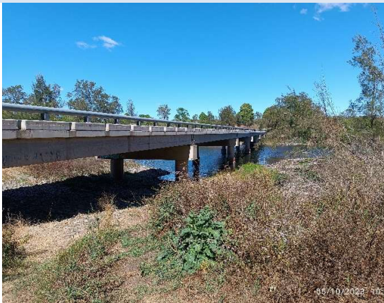
Photo 5: Turners Flat Bridge
