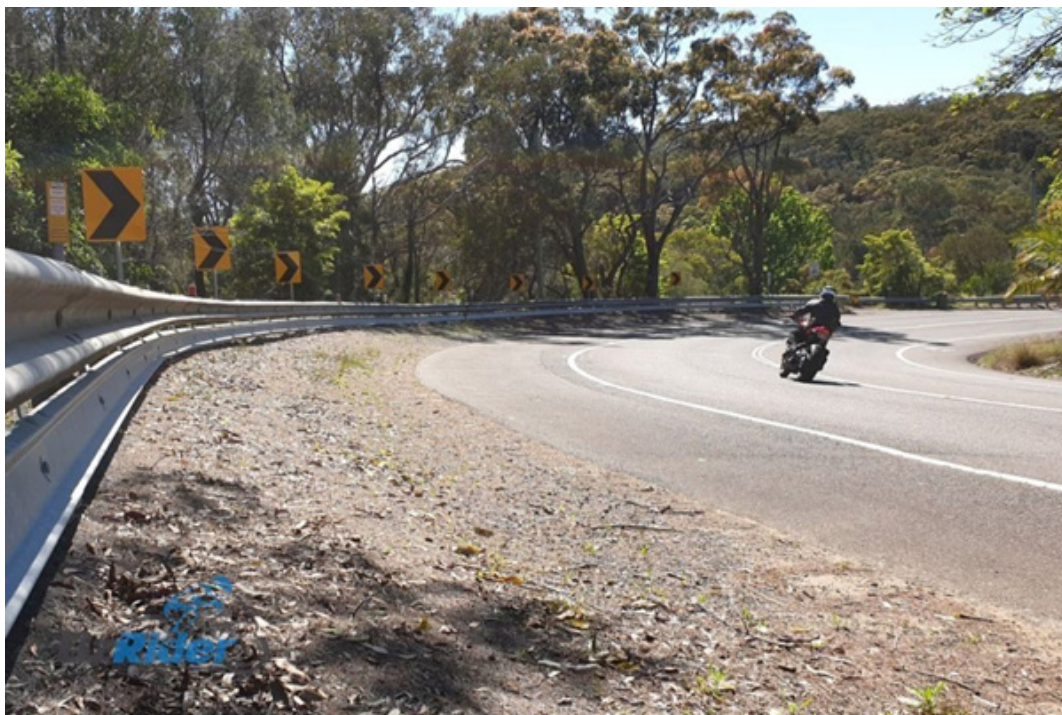
Figure 29: Safety Barrier with Rub Rail
