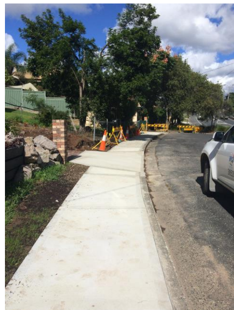
Lord Street, East Kempsey – Footpath Renewal
