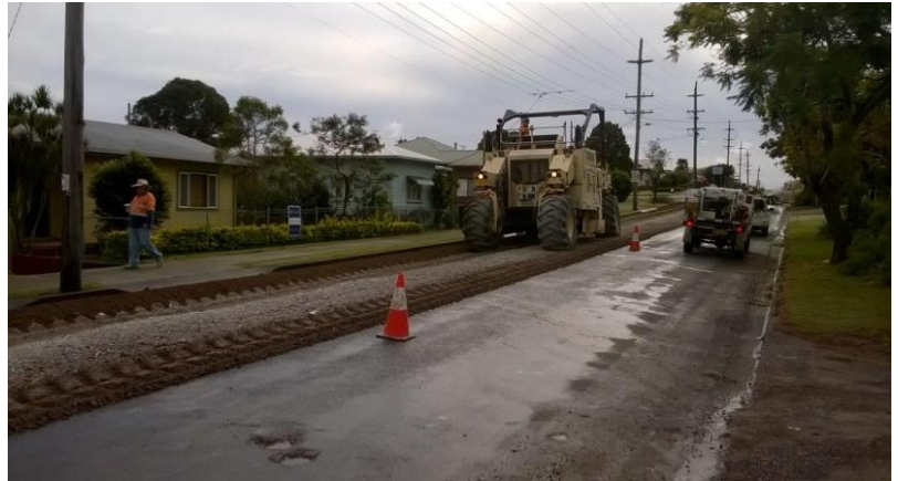
Recycling of existing gravel pavement via in-situ stabilisation with the addition of lime and/or cement. The old gravel and additional materials are mixed by a pulveriser and then re-compacted to reform the roadway
