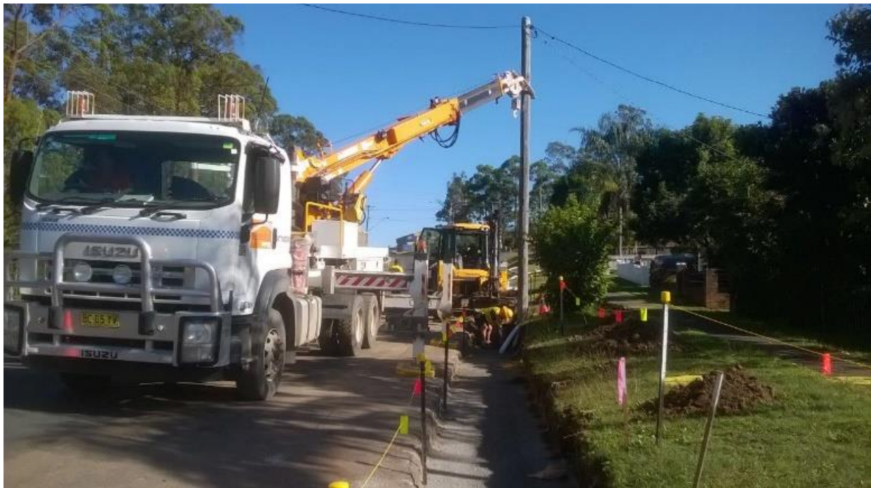
River Street, West Kempsey – rehabilitation from North Street to Jack Williams Crescent
