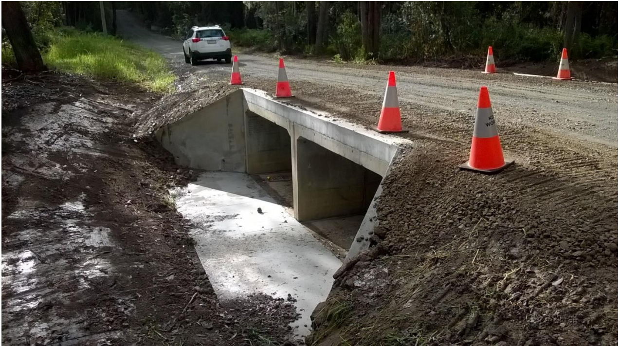
Lukes Lane culvert – installation of headwalls and aprons
