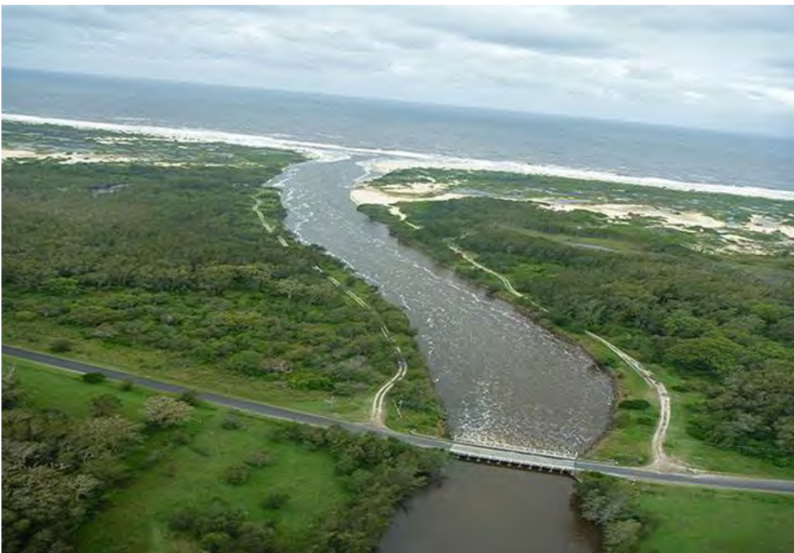
Figure 2-10 Ryans Cut - Ocean floodwater outlet discharging flood water from the Belmore area into the ocean, 2013 event (source: Kempsey Shire Council)
