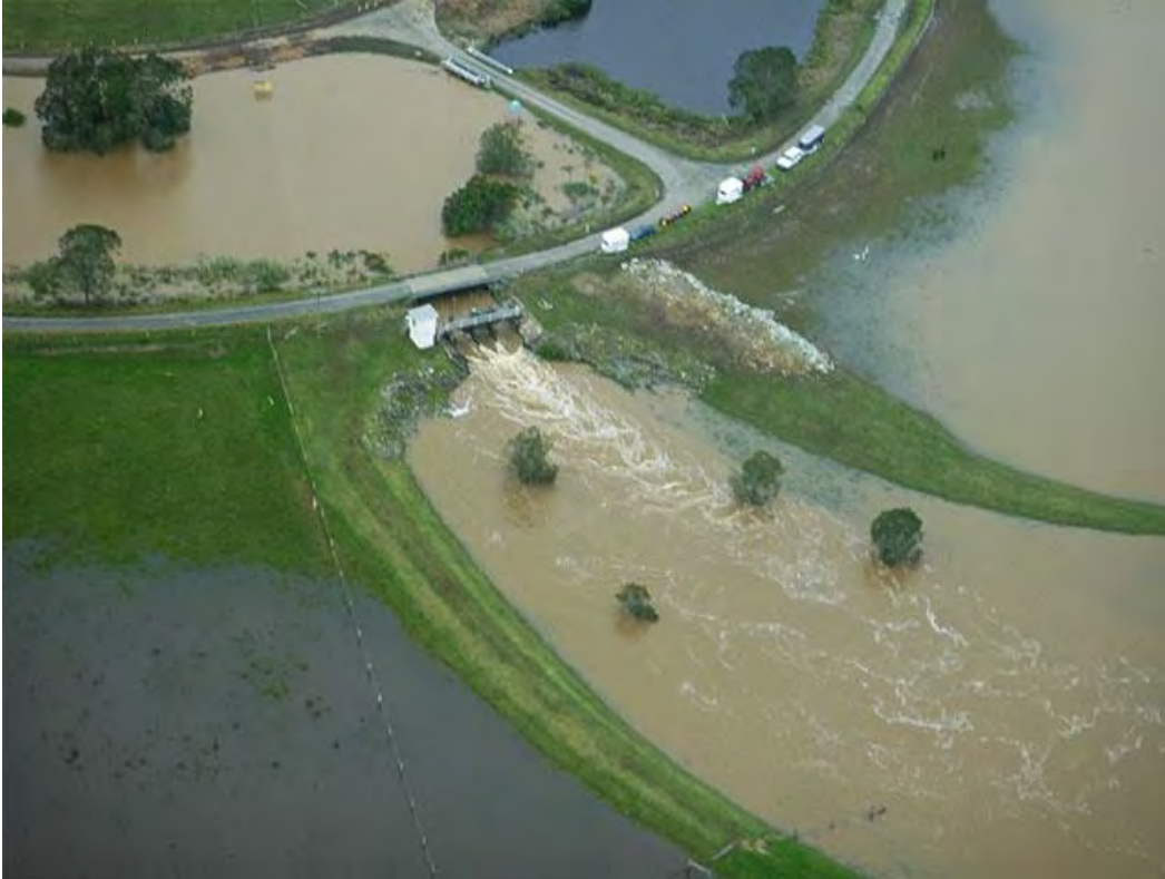
Figure 2-10 Ryans Cut - Ocean floodwater outlet discharging flood water from the Belmore area into the ocean, 2013 event (source: Kempsey Shire Council)
