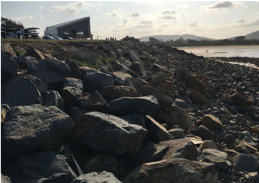
Existing erosion protection measures
