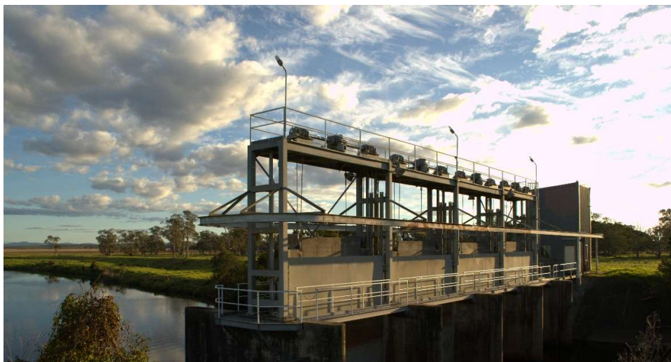
Belmore River Relief Floodgate Structure
