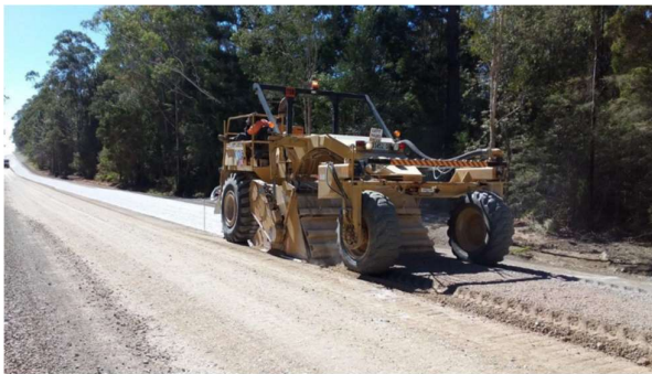
Pavement stabilisation with lime to recycle and strengthen the existing pavement material
