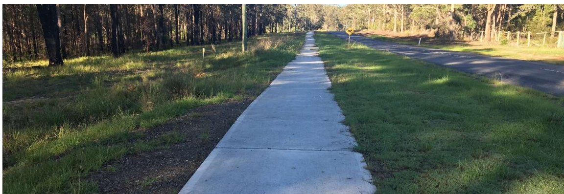
Gowings Hill Road footpath/cycleway
