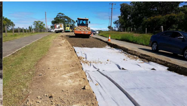
Excavation and replacement of inadequate pavement
