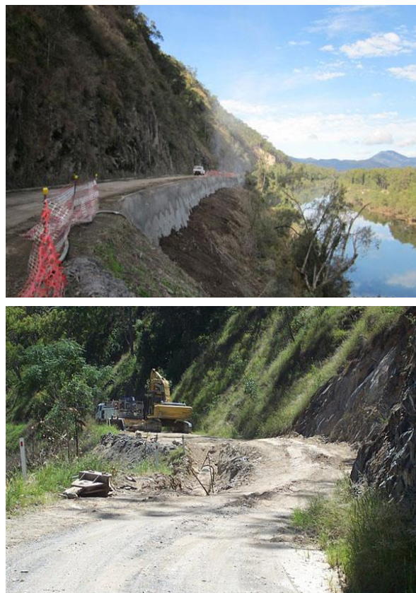
Figure 15. The Kempsey to Armidale Road
